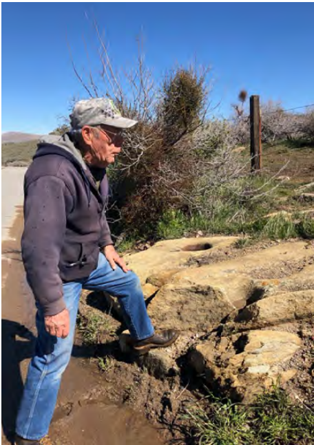
Buzz standing next to the ground stone mortars damaged by road crews in front of the Banner Queen Ranch in February, 2019
