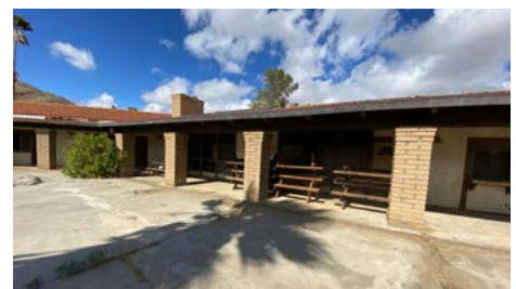
ABOVE TOP: Before clean-up at the Southern Heritage and Visitor Center CENTER: An almost full load going to the dump BOTTOM: Backyard patio after clean-up
