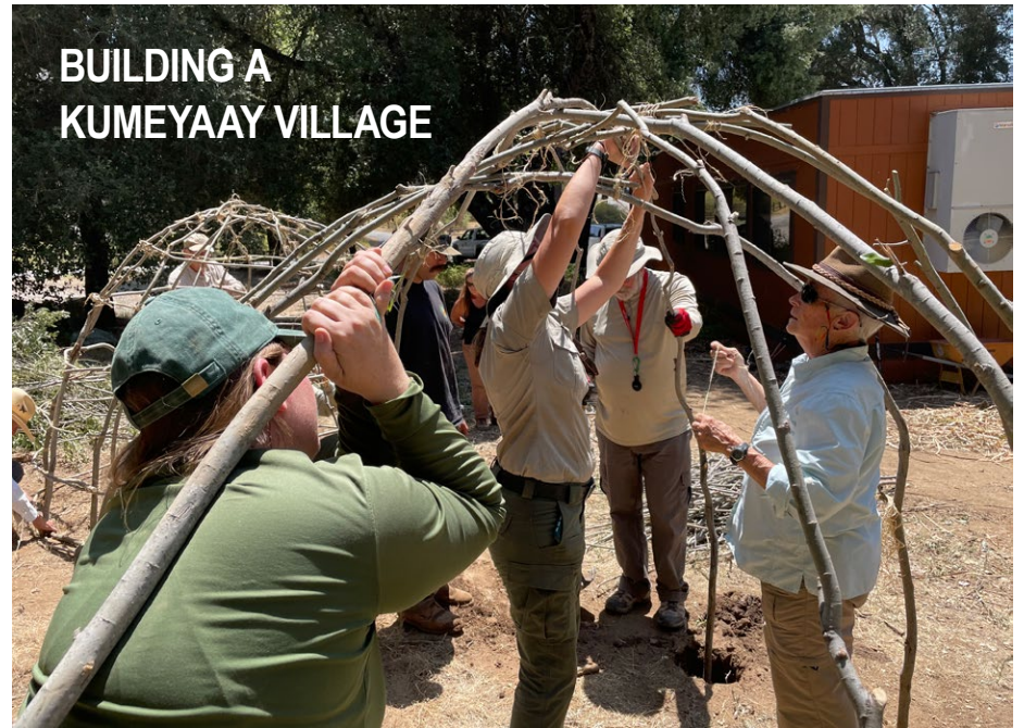
On August 18 and 19, volunteers help construct five e'waa structures (houses) under the direction of Kumeyaay Elder and educator Stan Rodriguez, PhD, at the Cuyamaca Rancho State Park. Associate State Archaeologist Hayley Elsken (front left) helps bend a willow branch so it can be tied with twine to create the frame. CDAS member Eugenie Newton (right) assisted. The village will be one of the topics covered by Dr. Rodriguez at the CDAS Kickoff meeting on October 23.
