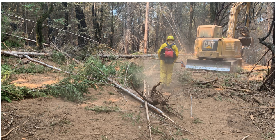
Repairing a dozer line in Fort Ross State Historic Park
